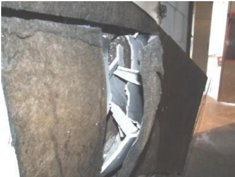
Core of the door leaf after removing of steel sheet from the unexposed door face.
