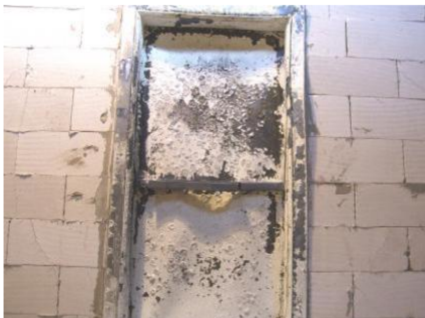
Exposed door face after the termination of the test.
